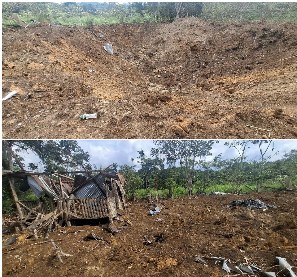
Two photographs of the damage caused to the property burned on March 1, 2026 and bombed on March 3, 2026. © 2026 Alliance for Human Rights
