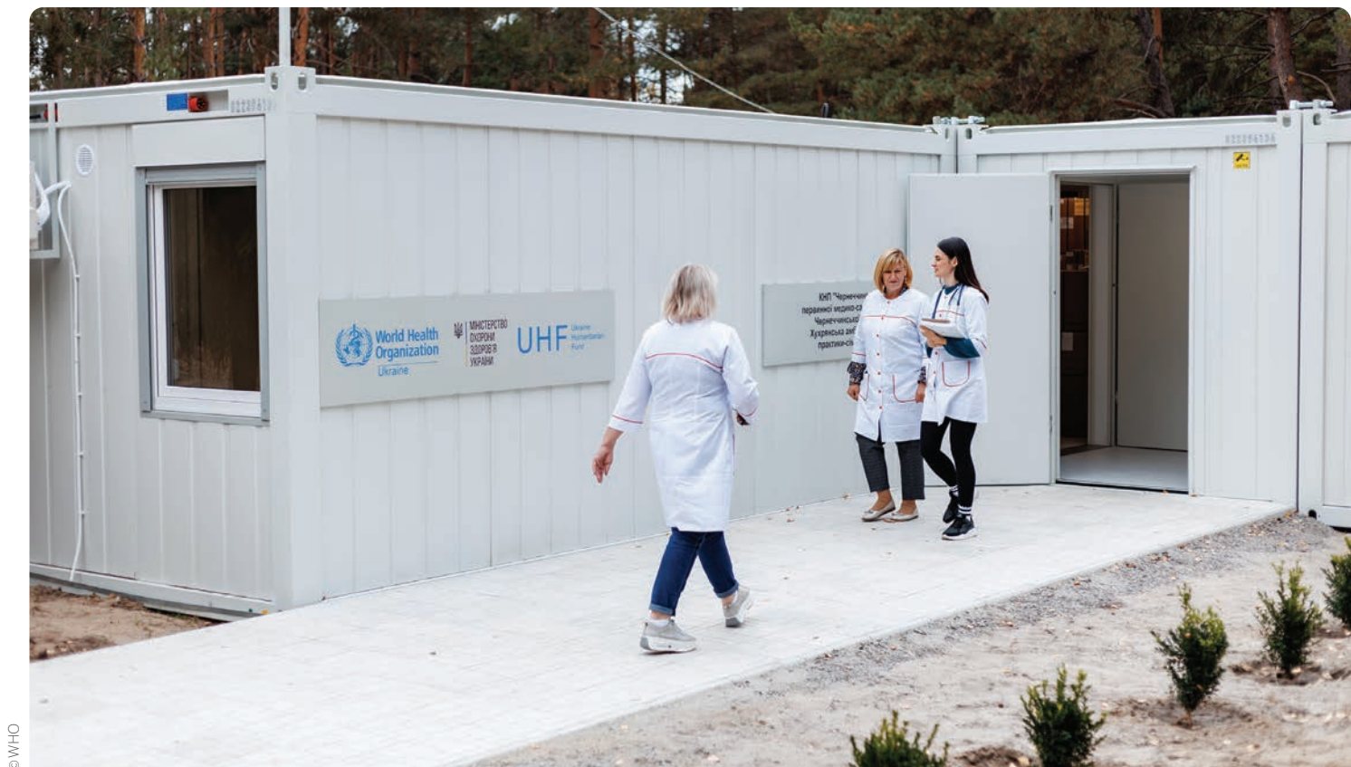
Primary prefabricated modular clinic in Sumy oblast, September 2025
