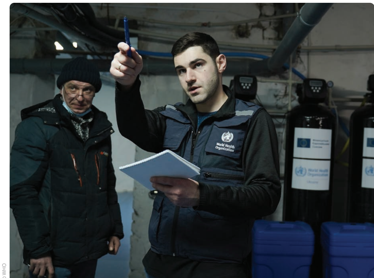
Installation of five water treatment stations in hospitals across Kharkiv city and oblast to ensure safe water access for patients and staff, Chuhuiv Hospital 2025
