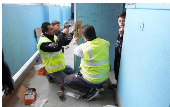
UNHCR partners carrying out shelter partitioning works inside a collective shelter to improve privacy and living conditions for displaced families. © UNHCR
