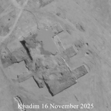
Figure 17.9 Status of GCS construction, Al Khadim
