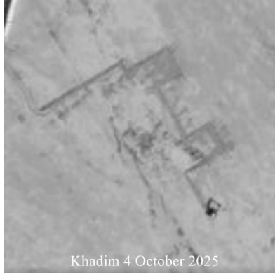
Figure 17.8 Start of GCS construction, Al Khadim
