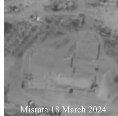
Figure 17.5 Start of GCS construction, Misrata
