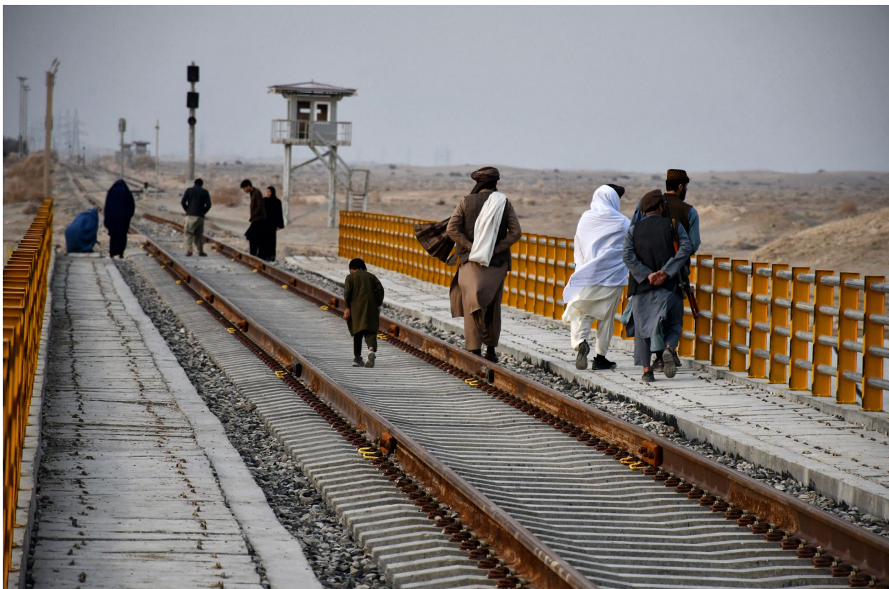
IEA security personnel walk along the railway tracks near the Qosh Tepa Canal in Hairatan, Balkh province, on the Afghanistan-Uzbekistan border.
