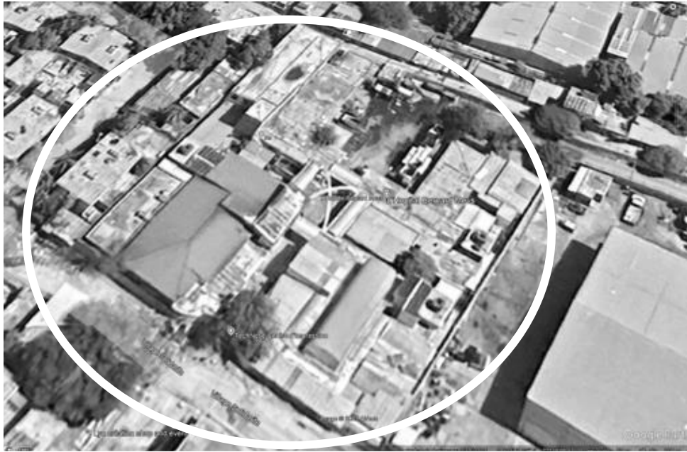
Figure 2. Bernard Mevs Hospital satellite image taken 15 March 2025.
