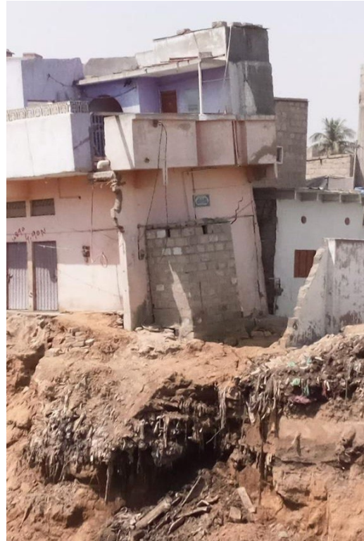
A house dangerously tilted due to landslides caused by excessive digging near a portion of a stormwater channel in Karachi, 2022. Residents claimed that authorities did not construct protective walls around demolished houses before beginning work on the stormwater channel. © 2022 Karachi Bachao Tehrik
