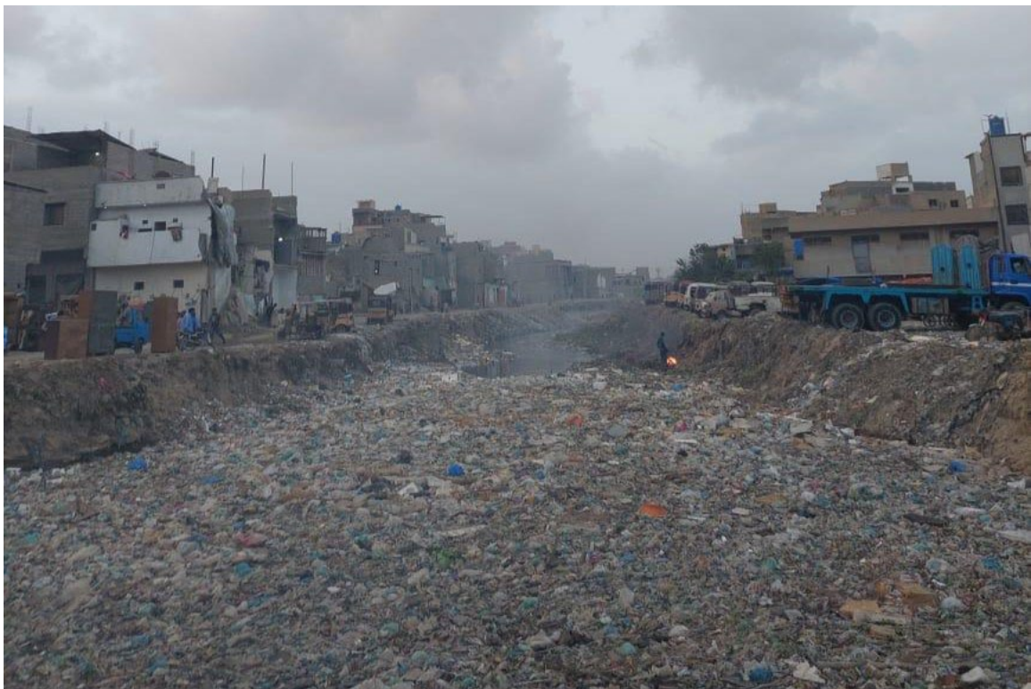
A section of a stormwater channel in Karachi clogged with solid waste, where authorities' claimed that rainwater could not pass through due to “encroachments.” © 2021 Karachi Bacaho Tehrik
