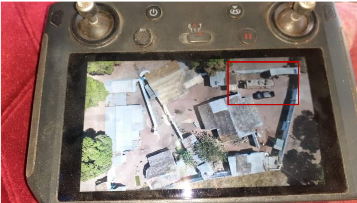
Annex 23: Drone image of the compound formerly belonging to Mahamat Al-Khatim with a “Chekan” type vehicle parked inside
