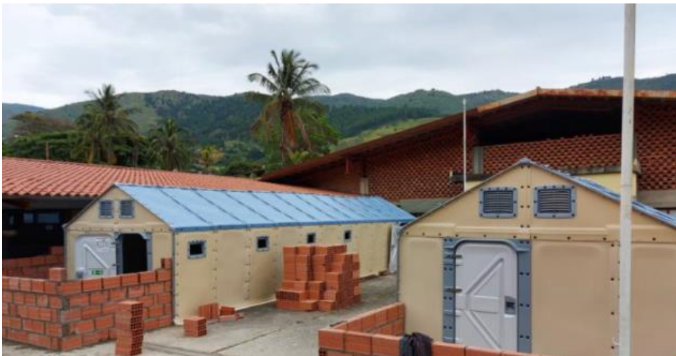
Emergency Shelter provided by UNHCR in Tovar Municipality, Mérida State, Venezuela. © UNHCR Venezuela
