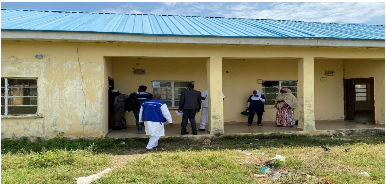
One of the 4 Blocks containing 16 units of staff quarters requiring urgent renovation
