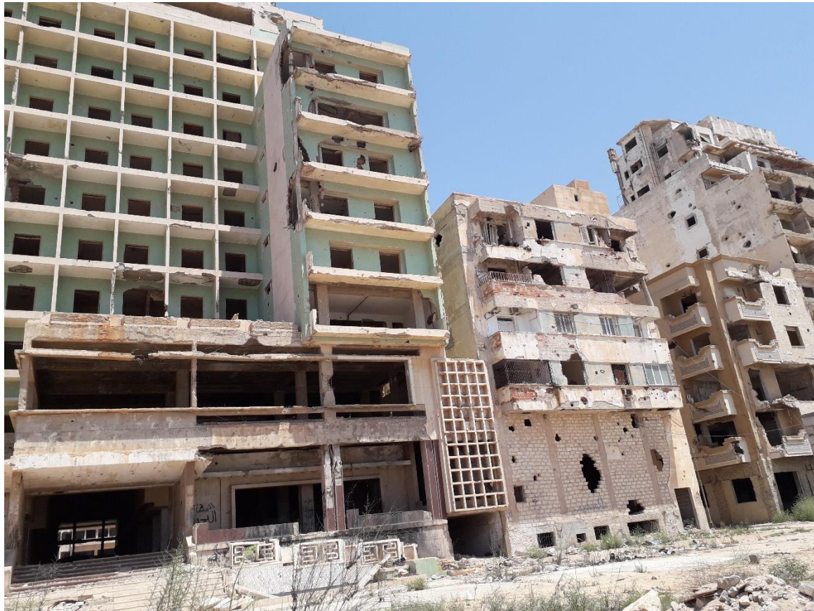
Damaged housing in the Al Sabri neighborhood, Benghazi (UNHCR)
