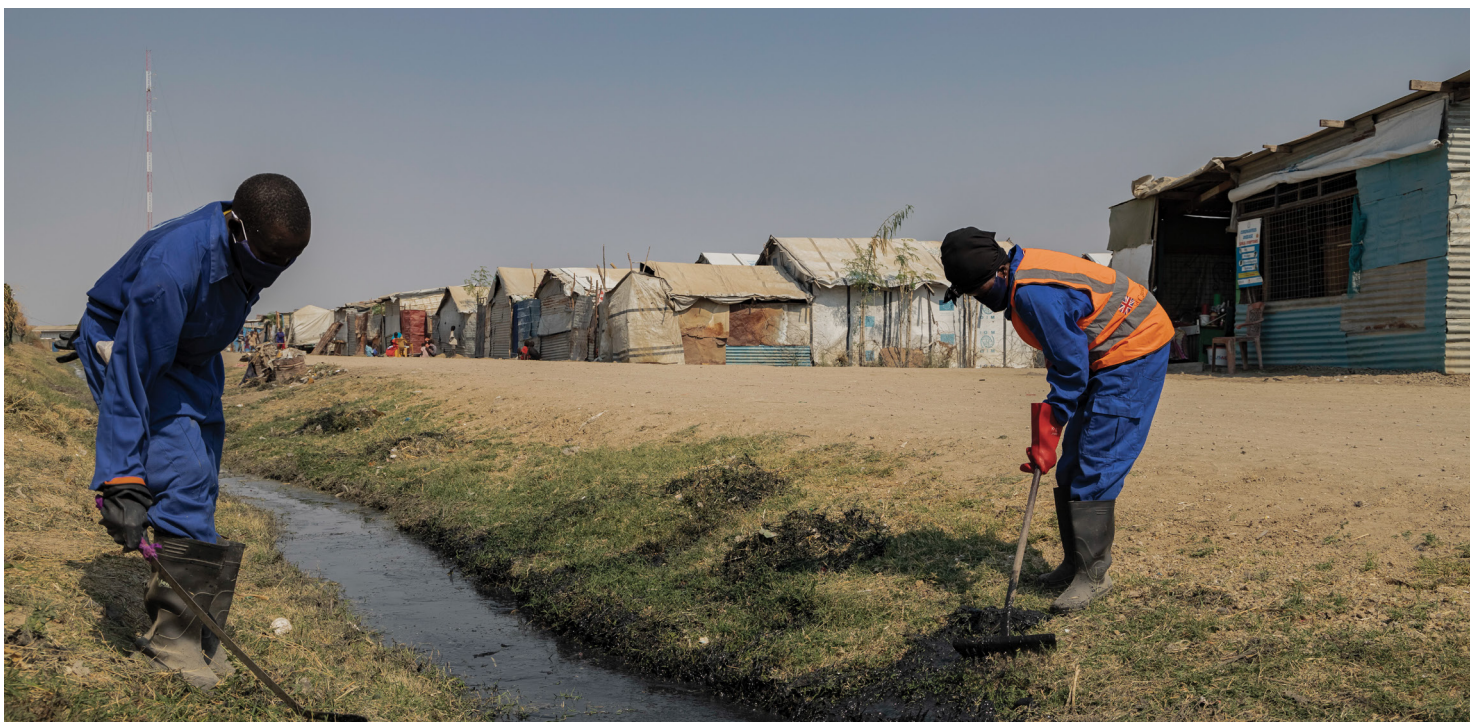
Drainage cleaning at Malakal PoC © IOM 2021
