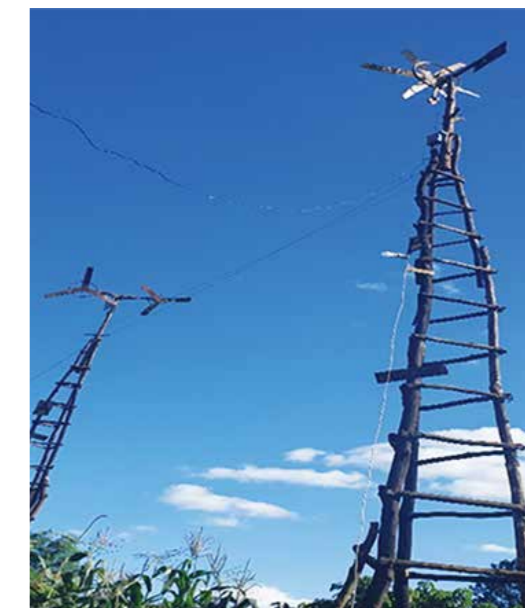
Power lines for the mini-grid installed in the community to increase power generation capacity for the rural population from 379 kW in 2019 to 385 kW in 2020. Rural communities have access to electricity for improved wellbeing and local economic activities to support livelihoods. Photo: UNDP Malawi.
