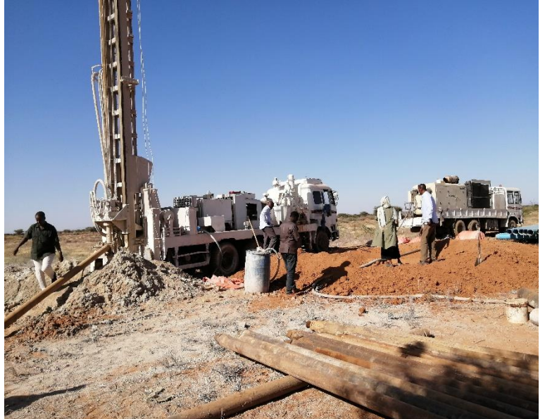
NRC drilling a borehole in IDP site in Burao Togdheer. Photo: OCHA
