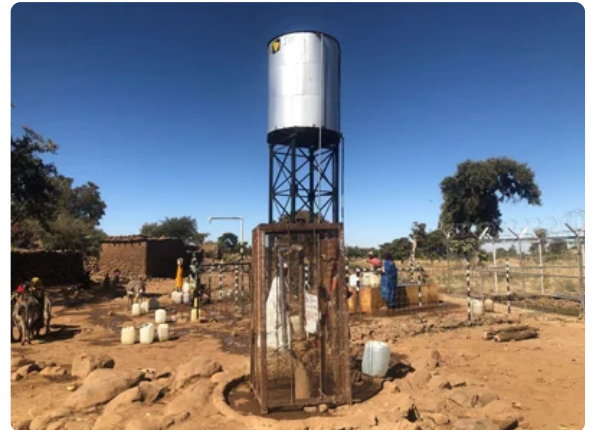
Solar powered mini-water yard upgraded from a hand pump by TGH with SHF funds (OCHA, January 2020)
