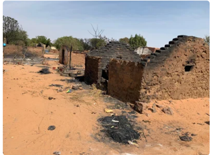
Destruction of homes in Krinding IDP camp, West Darfur (UN, January 2020)
