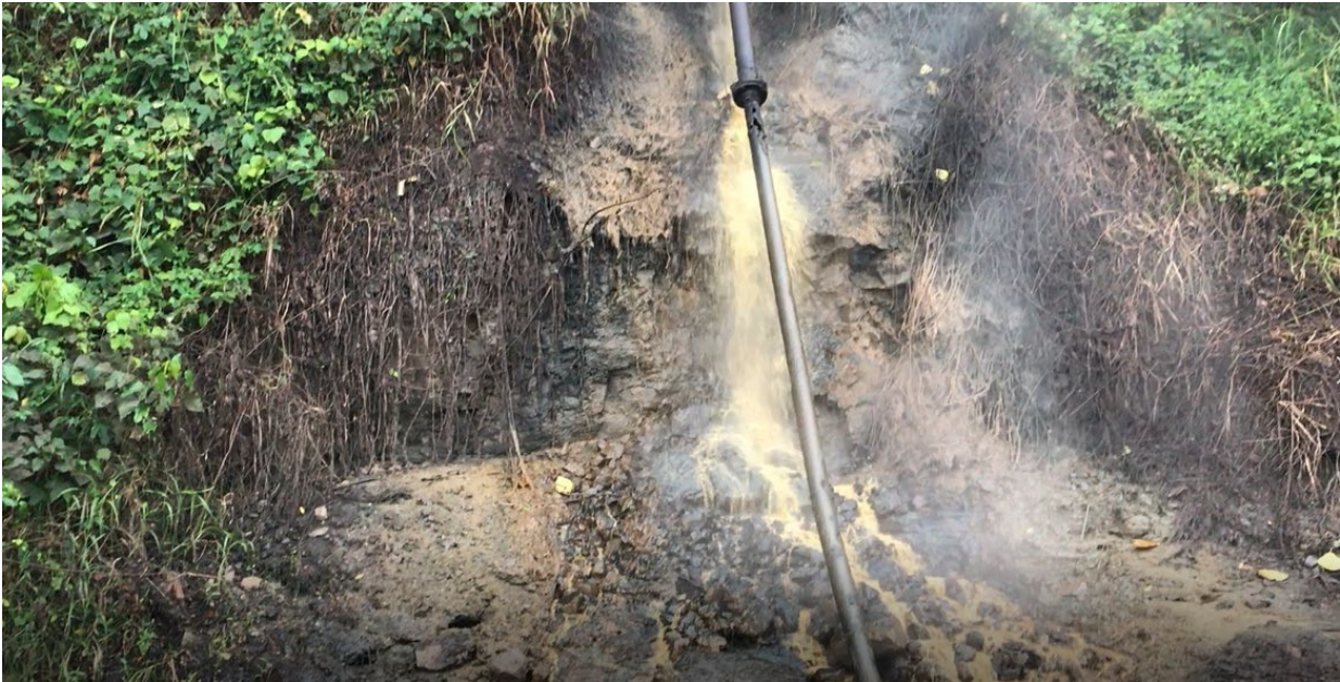
The Lokutu mill pipeline is located to the west of the mill, facing the Congo River. In the picture above, a leak in the pipeline releases some of the mill's effluents onto the riverbank.
