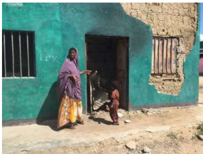
Figure 4 Hawa Abdullahi in front of her damaged house. Photo Credit: OCHA/Jodri
