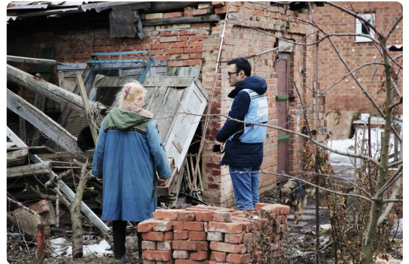
Valentina is showing her damaged house in Sloviansk, Government-controlled area of Donetsk oblast. After Valentina's house was shelled twice, only two walls remained standing. OCHA/I.Grishko/2019
