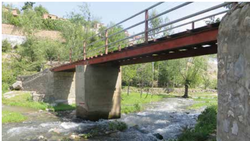
CERP-funded pedestrian bridge in Kabul. (SIGAR photo)
