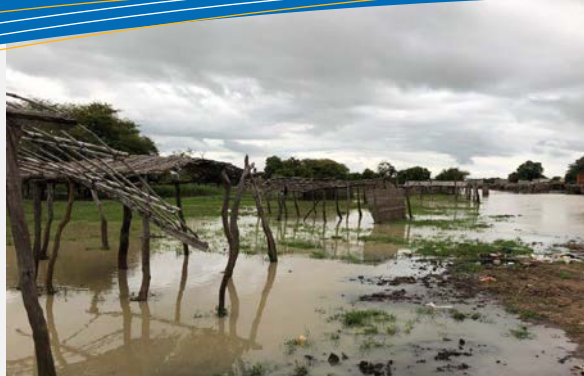
Heavy rains and flash floods destroy many structures in Um Dukhun, Central Darfur (UN, Sept 2018)
