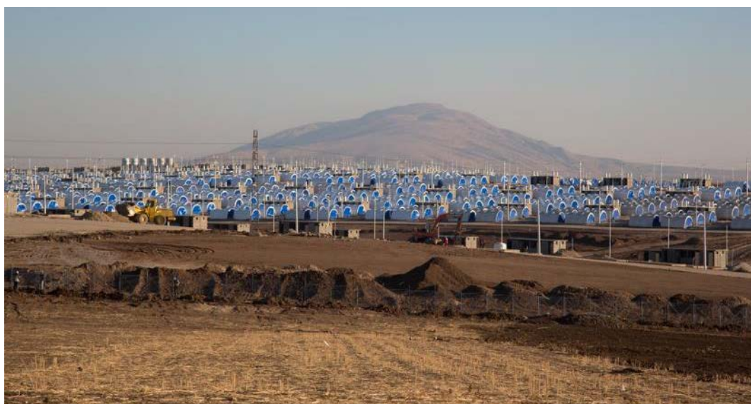
Nargizlia Camp, northern Mosul, under construction. Credit: OCHA/Elias
