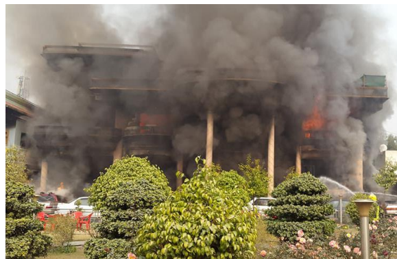
During the fighting, a building of SCA in the neighbouring compound caught fire. Photo: SCA
