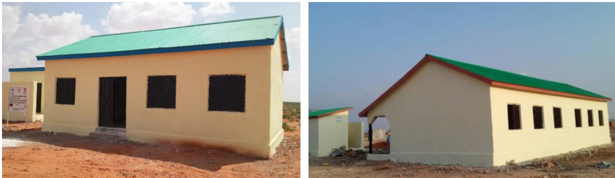
One of two newly constructed community centre [left] and school [right] along with latrines in Galkacyo for returnees and host community. © NRC/Galkacyo, November 2017
