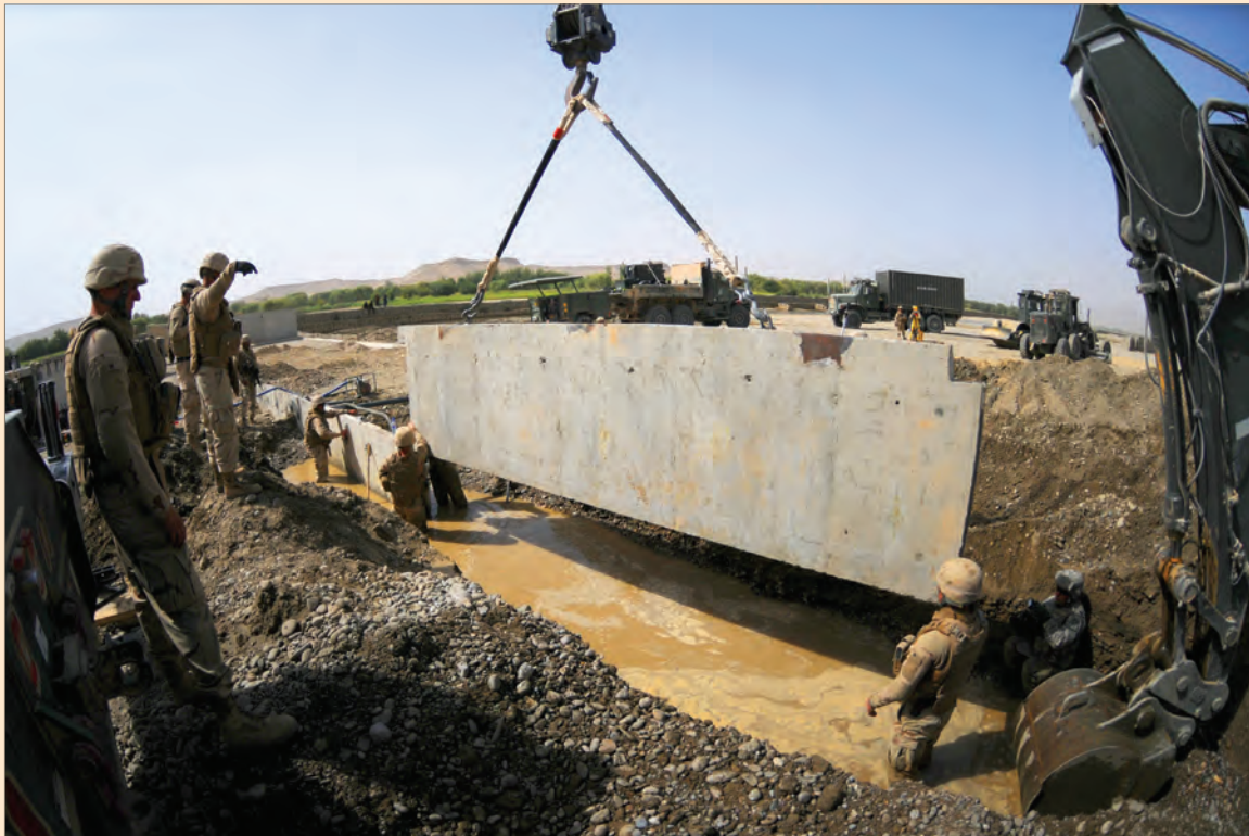
U.S. Seabees place prefabricated concrete pieces in the riverbed at the Musa Qal'eh low-water-crossing project. (Navy Photo by Mass Communication Specialist 1st Class Russ Stewart)
