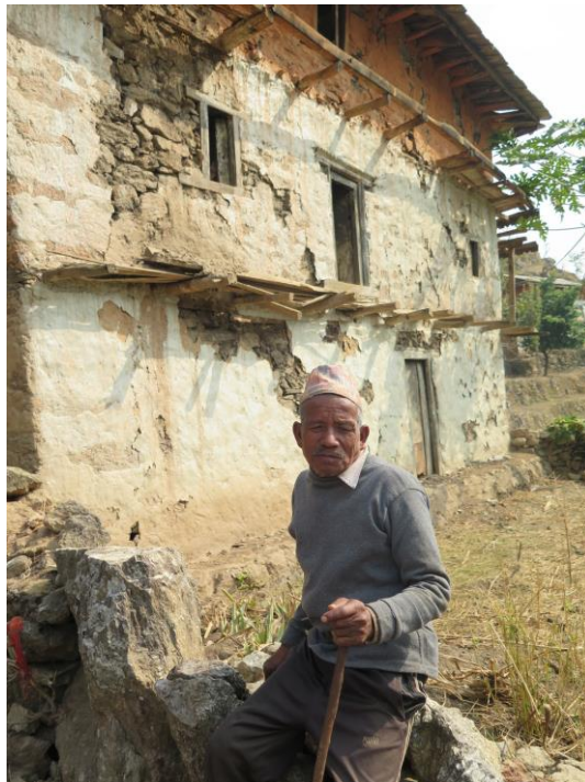
Nur Bahadur Maji sits in front of his damaged house in Dolakha district. ©Amnesty International
