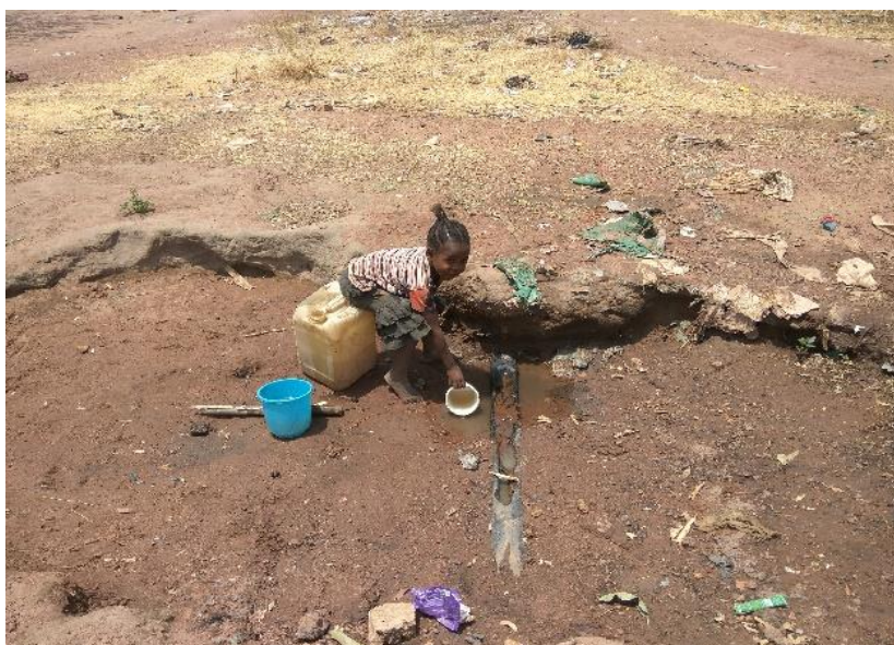
@UNICEF South Sudan 2017: A child collecting water from a damaged water pipeline in Yambio town.
