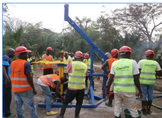
©VWW. Kouango, Ouaka Prefecture – Workers renovate drilling equipment with the help of the "Village Drill" innovative technique.
