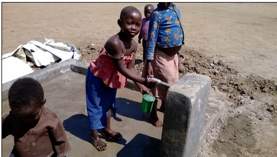
Congolese refugee children use a recently installed water station at the Child Friendly Space in Bubukwanga transit centre. ©UNHCR/A.Ndungu
