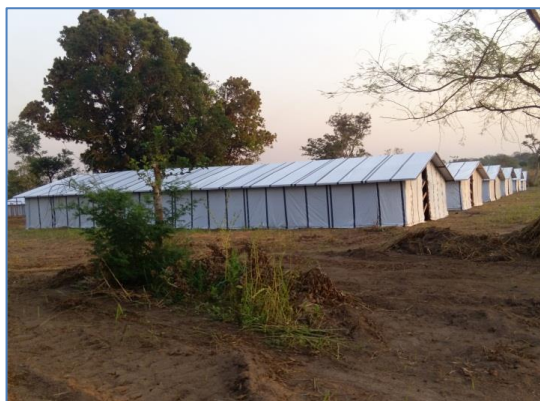
Set-up of community shelters at the "Lazare" site. ©OCHA
