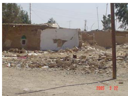
Destroyed House in Al Tash Camp - UNHCR
