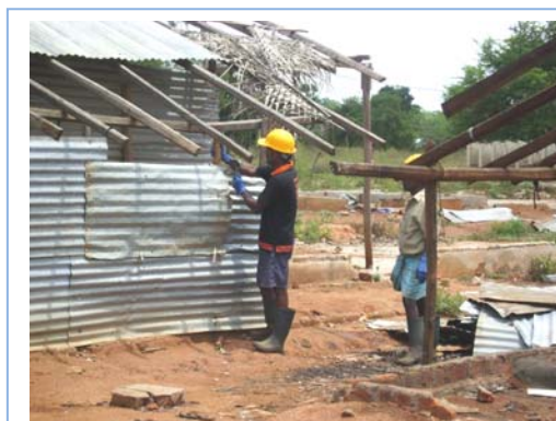
Photo 12: Shelter maintenance work in Zone 0; Credit: UNOPS
