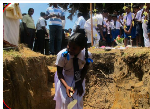
Photo 4: Student representative laying the foundation for Mullaitivu Maha Vidyalayam; Credit: UNICEF
