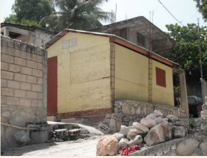
Transitional shelter (“T-Shelter”), Port-au-Prince, summer 2012. Photo credit: Laura Wagner.
