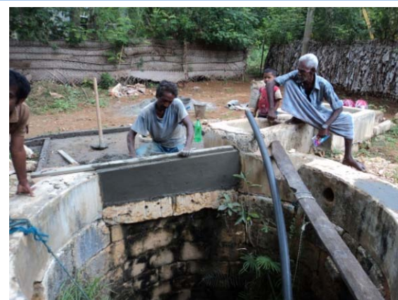
Photo 6: Dug well rehabilitation in Jaffna. Credit: UNICEF
