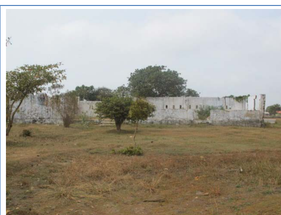
Photo 1: Thanankkilappu GTMS in damaged condition Credit: UNICEF
