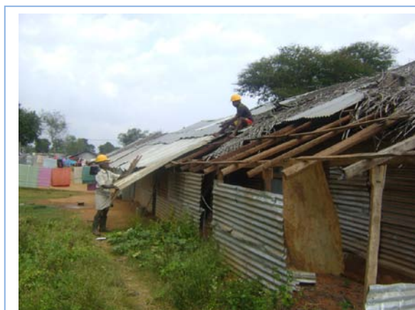
Photo 4: Emergency Shelter roof repairing in Menik Farm Zone 0 Credit: UNOPS
