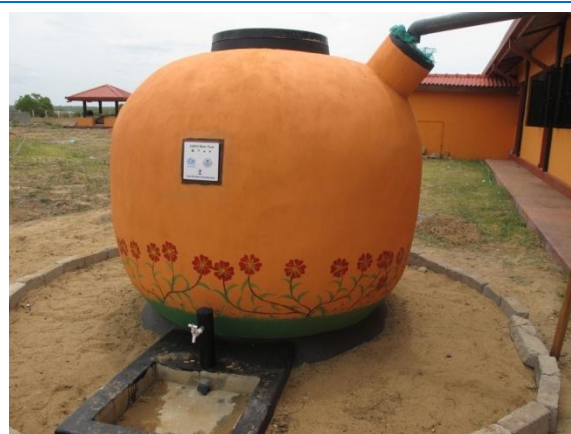
Photo 7: Rain Water Harvesting System implementation, Credit: UNICEF
