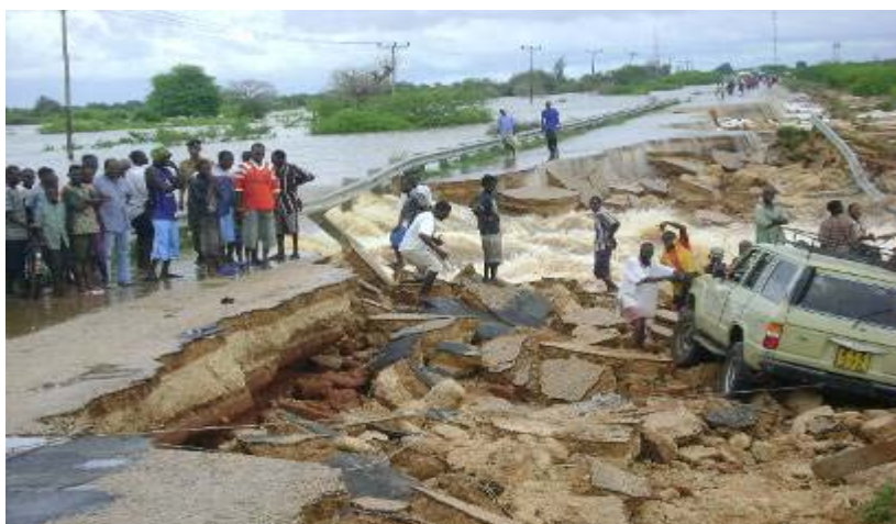
The road to Tana Delta (Garsen), Hola and Lamu is cut off after heavy rains. Photo: KRCS Malindi
