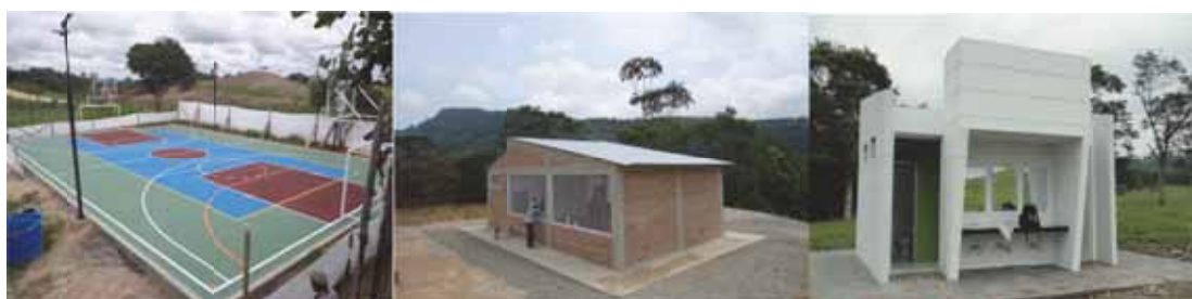
Sample of communal works of the Quick Response Programme of the Special Administrative Unit for Territorial Consolidation of the Government of Colombia: communal rooms, sports settings and sanitary batteries (Norte de Santander and Caquetá)
