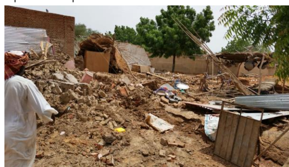
Houses damaged by flooding in En Nuhut locality, West Kordofan State. (OCHA, 2016)
