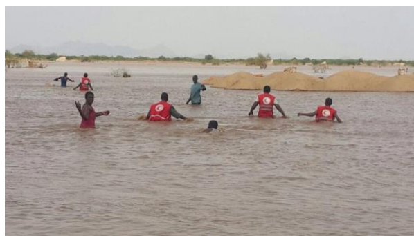
Construction of a barrier in a flood-affected area of Kassala State. (SRCS, 2016)
