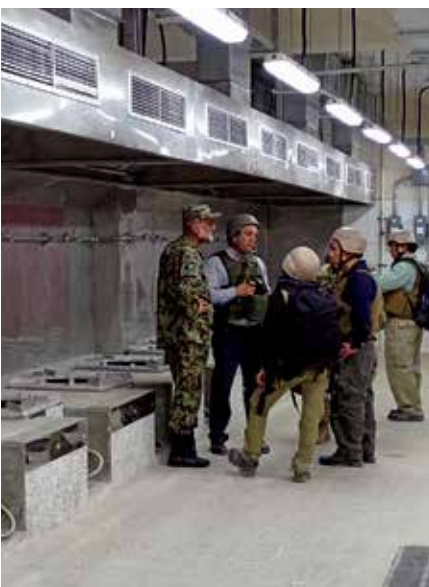
SIGAR inspects kitchen facilities at the Kabul Military Training Center. (SIGAR photo)
