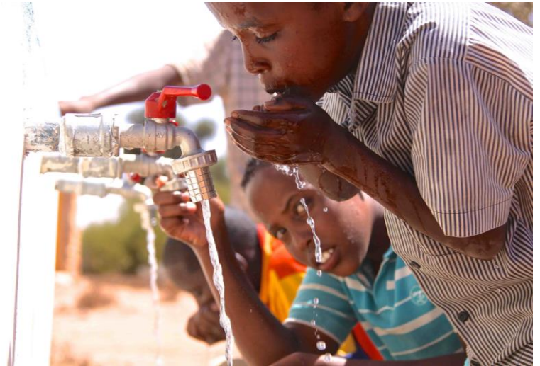
Newly installed water point in Somaliland. Credit: UNICEF/Makundi
